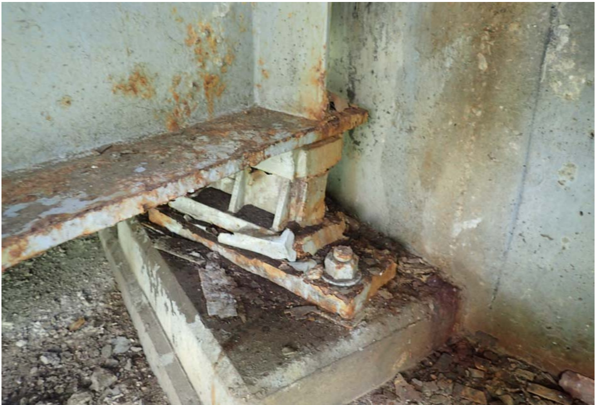
View of the downstream bearing at abutment 1.
