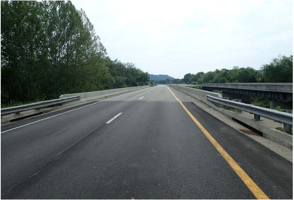
Approach to abutment 1.
