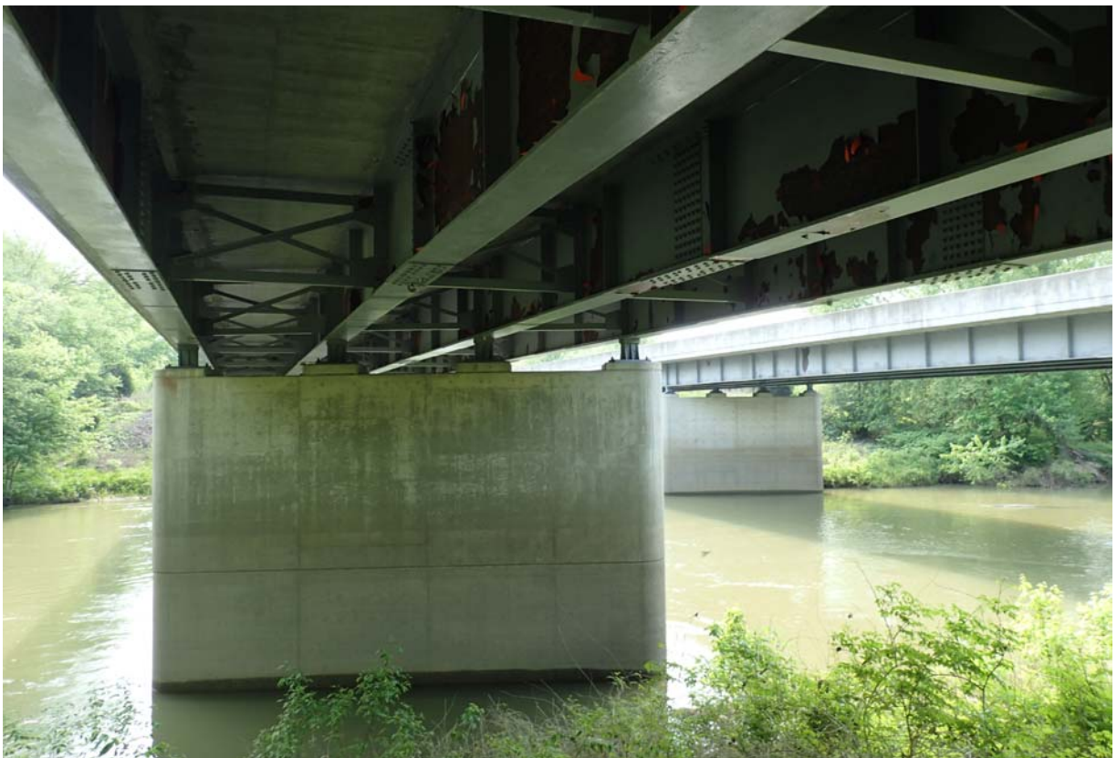
Typical view of span 1 and pier 2.
