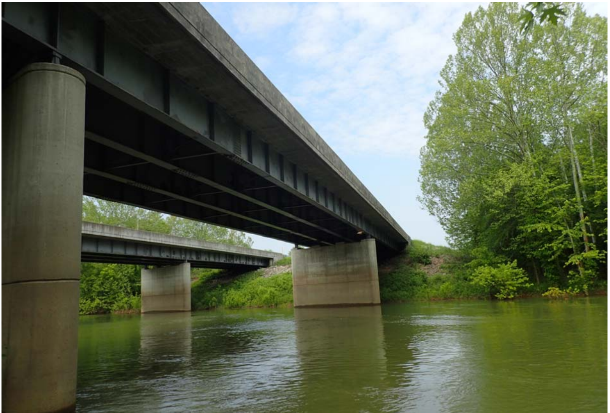
Typical view of span 2 and pier 2 from downstream.
