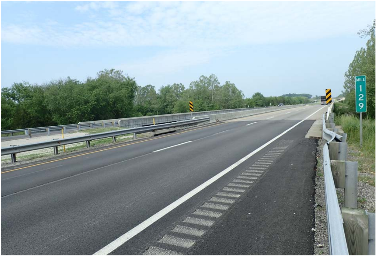
Approach to abutment 4.
