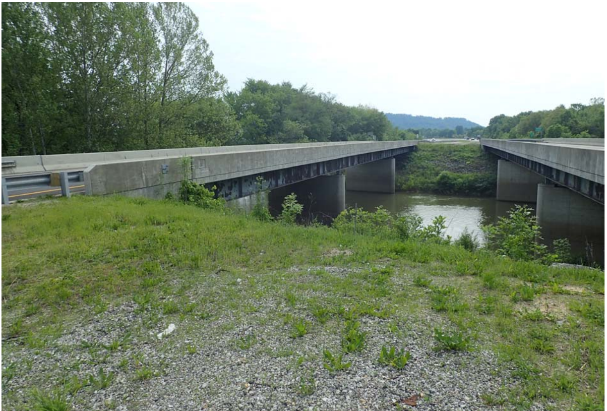
View from upstream near abutment 1.
