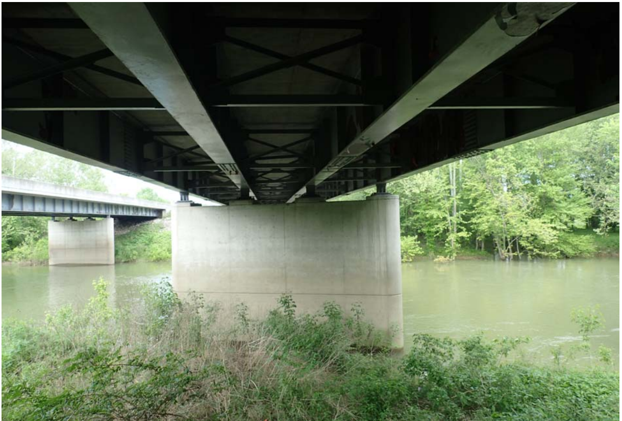
Typical view of span 3 and pier 3.
