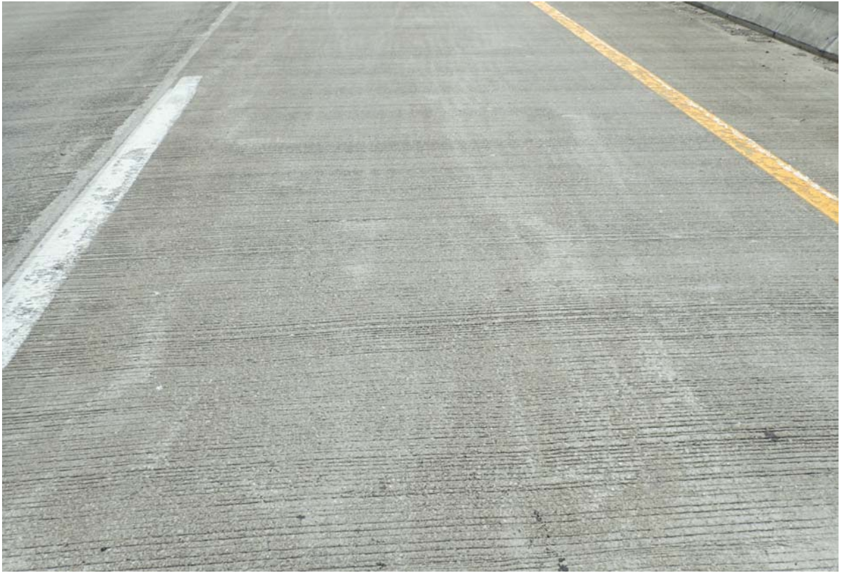
Typical view of the wearing surface near abutment 1.
