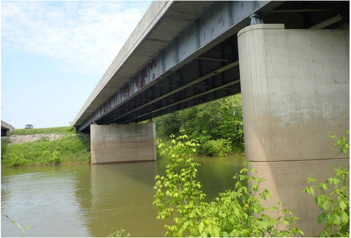
Typical view of span 2 and pier 2 from upstream
